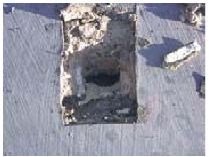
Photograph 6-Void under insulation at ridge
