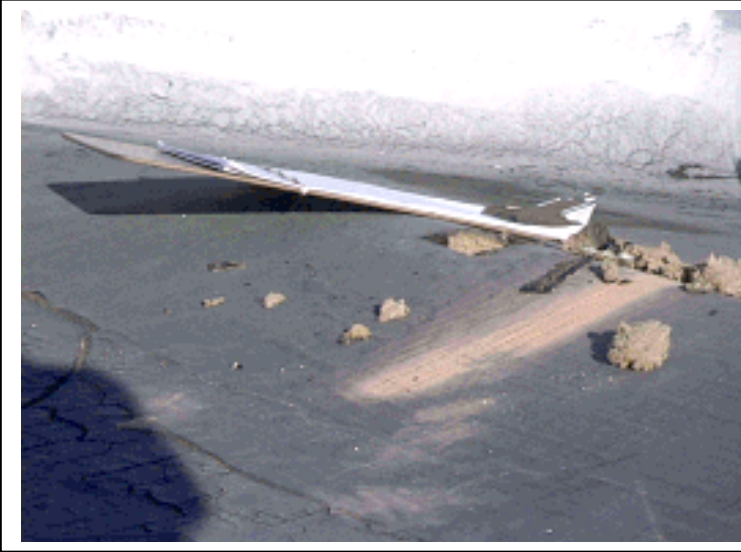
Photograph 5-Ridge in insulation
